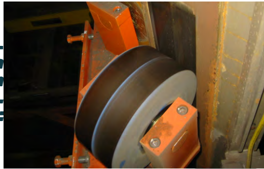
Floor-to-floor elevator guide wheel of NYTEC-HS
